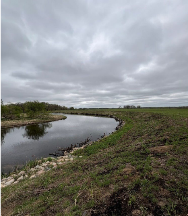
Streambank stabilization at the Crane Meadows Wildlife Refuge (Morrison County, MN)
