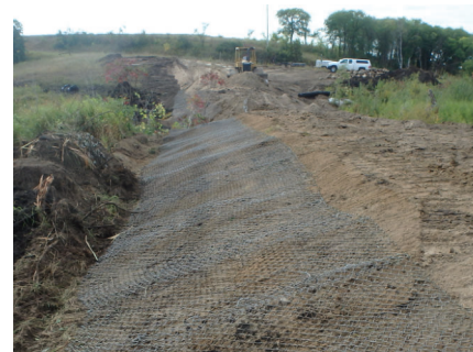
Left: Cattle graze on a recent tree removal/wetland restoration site. Right: welded wire going in on the front slope of a ditch plug. The wire protects the structure from muskrat use and therefore potential structure failure, ensuring the wetland is restored for the long term.
