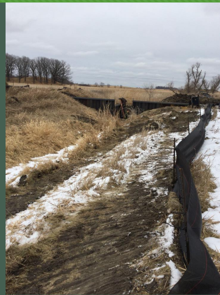
Sheet Pile Wier Installation
