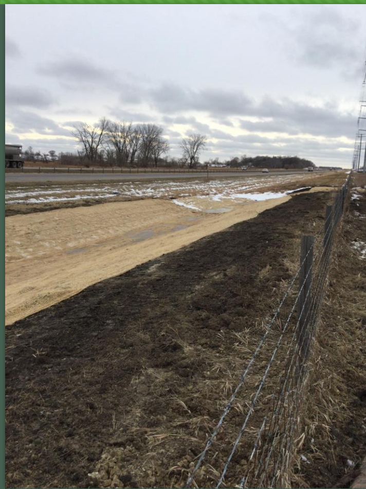
Erosion Controlled Diversion along I94
