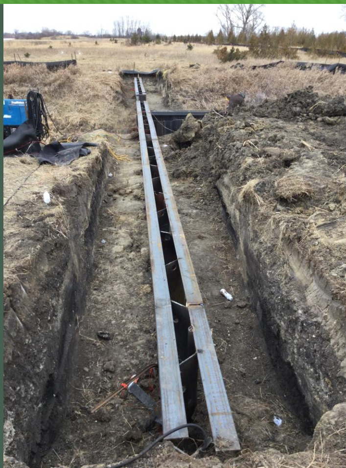
Sheet Pile Wier Installation
