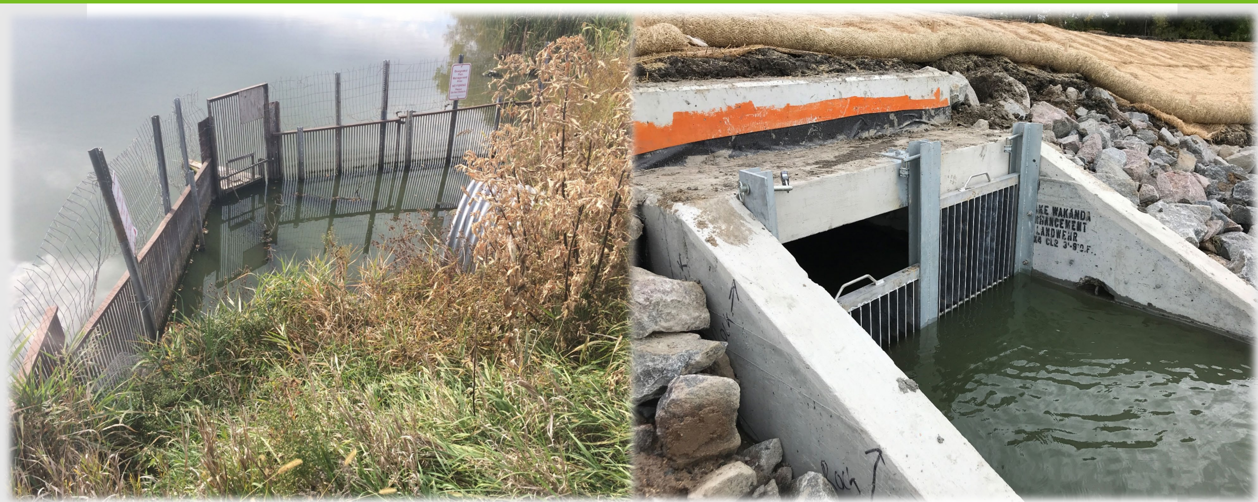
Replaced a large CMP culvert with a 4x6 concrete box and 2 removable screens. Located on County Road 123
