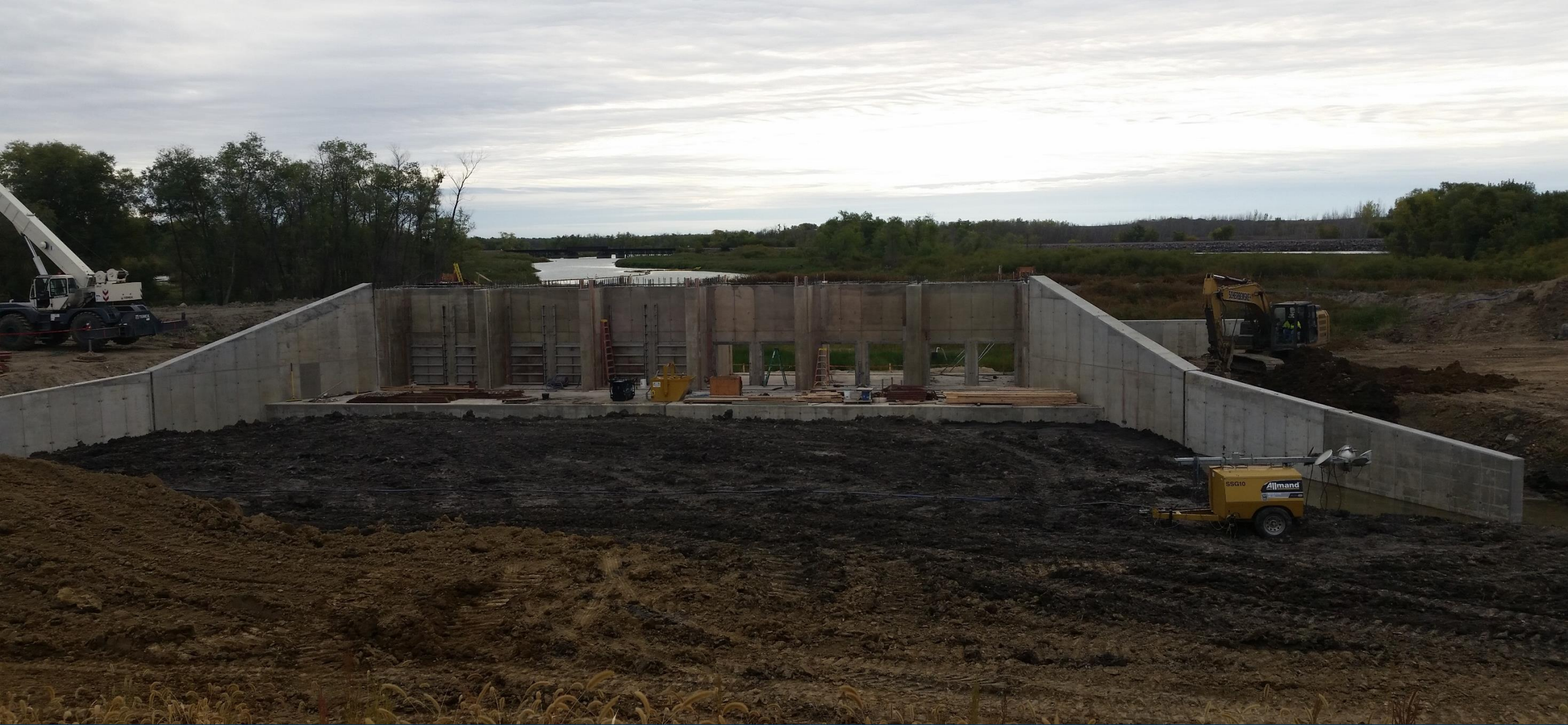
Water control drawdown structure in progress
