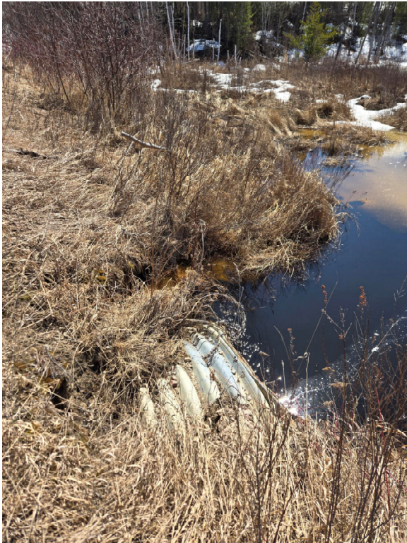
Above: One of the 16 culverts identified causing bank erosion and sediment loading in the watershed.
