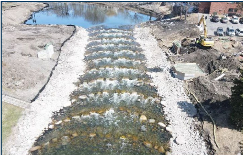
Picture 4. DNR and Cottonwood Co. SWCD propose replacing the current dam with a rock arch-rapids and variable crest water control structure to improve fish passage and habitat in Talcot Lake.
