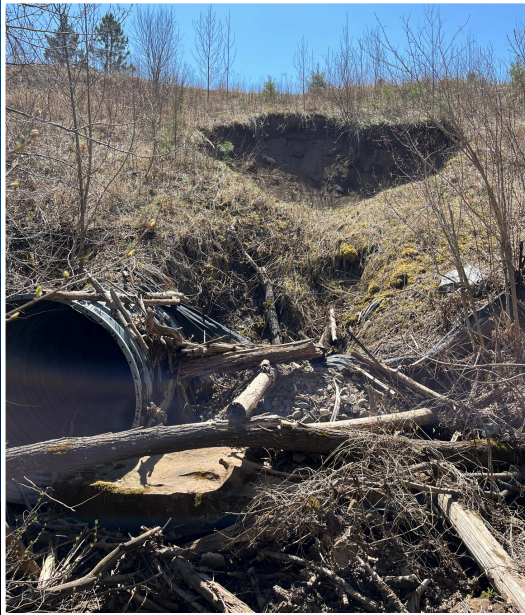
Culvert failure and embankment instability along the Munger Trail.
