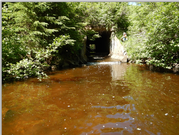
Above: Views looking upstream (left) and downstream (right) demonstrate that the culvert is undersized and does not meet the bankfull condition of the Little Devil Track River.
