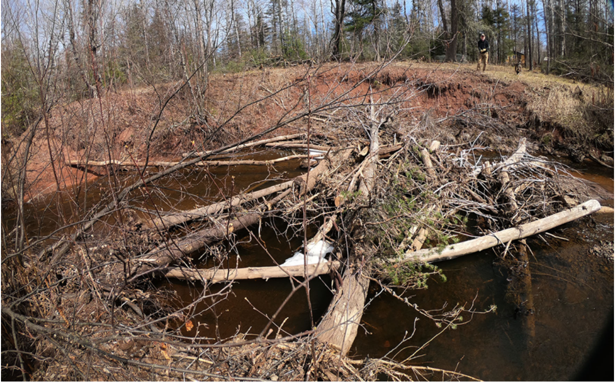
Reach 8 bank stabilization: Note the raw clay bank discharging sediment to the stream. This project will restore the spawning habitat at the tail end of the pool and provide instream overhead cover for juvenile rearing habitat.
