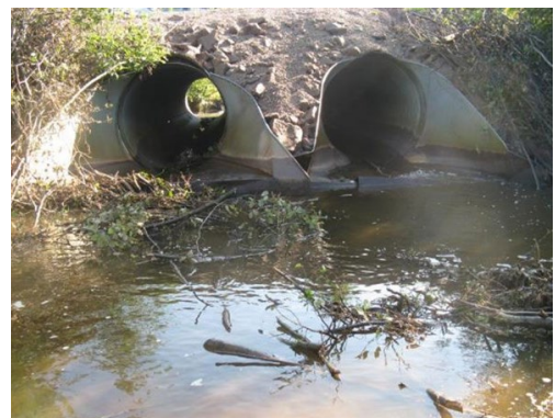
Culvert before modification:
