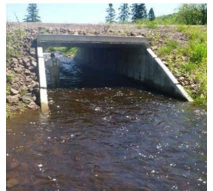
Culvert after modification:
