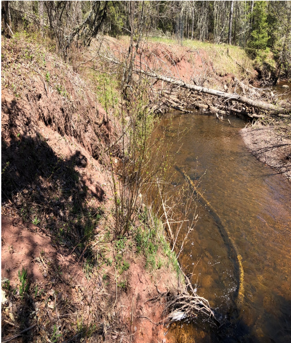
Reach 8 Bank Slumping
