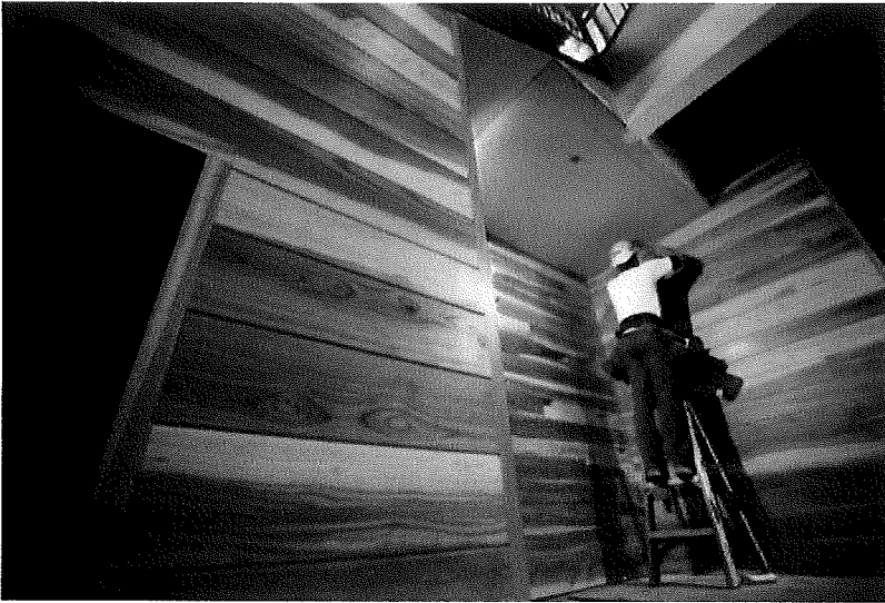
Utilization of wood from felled ash trees in Eagan's Public Safety Center (Photo from Brian Peterson, Star Tribune)
