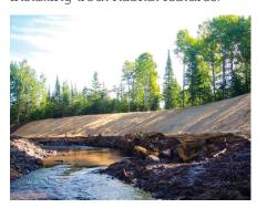
The creation of these new stream features allows the floodwaters to crest the new streambank instead of eroding the face of an unstable slope. The result is a stream with a narrower and deeper channel. This new channel design transports sediment to maintain deeper pools, which ultimately provide significantly better trout habitat
