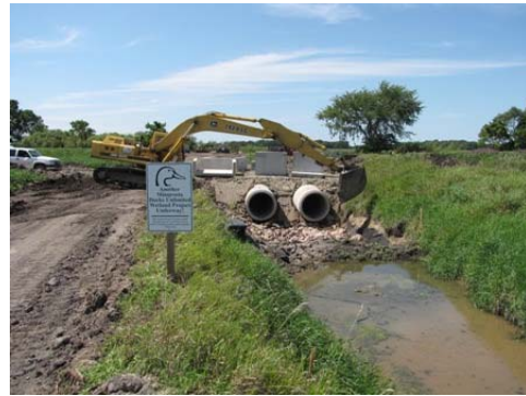
Ongoing construction of culvert at Rice Lake
