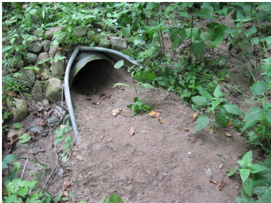
Photo 1 Culvert off-site to the west, carrying sediment from housing.
