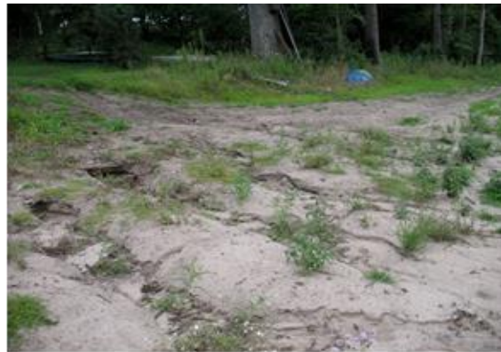
Photo 4: Rill erosion at lakeshore/lawn edge.
