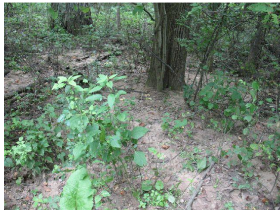
Photo 2 Sediment outwash from culvert covering ground.
