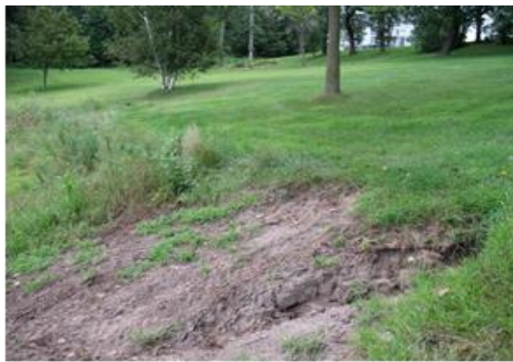
Photo 3: Erosion at lakeshore/lawn edge.
