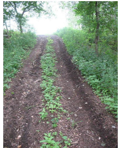
Photo 5: Truck track on south edge of Lake; entrenched and erosive.
