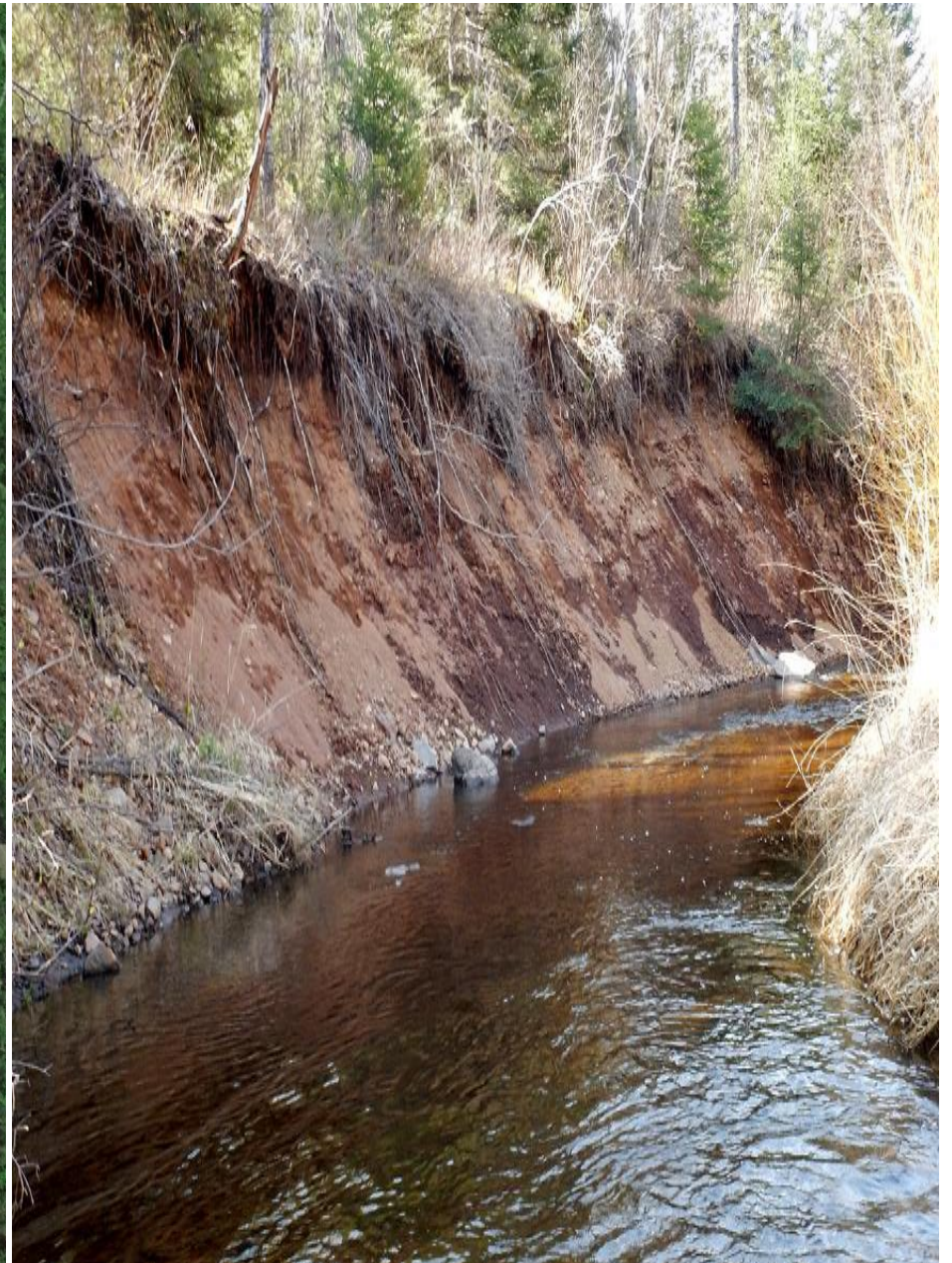
Slumping Bank Lower Reach 4 – Rehabilitation similar to Reach 12
