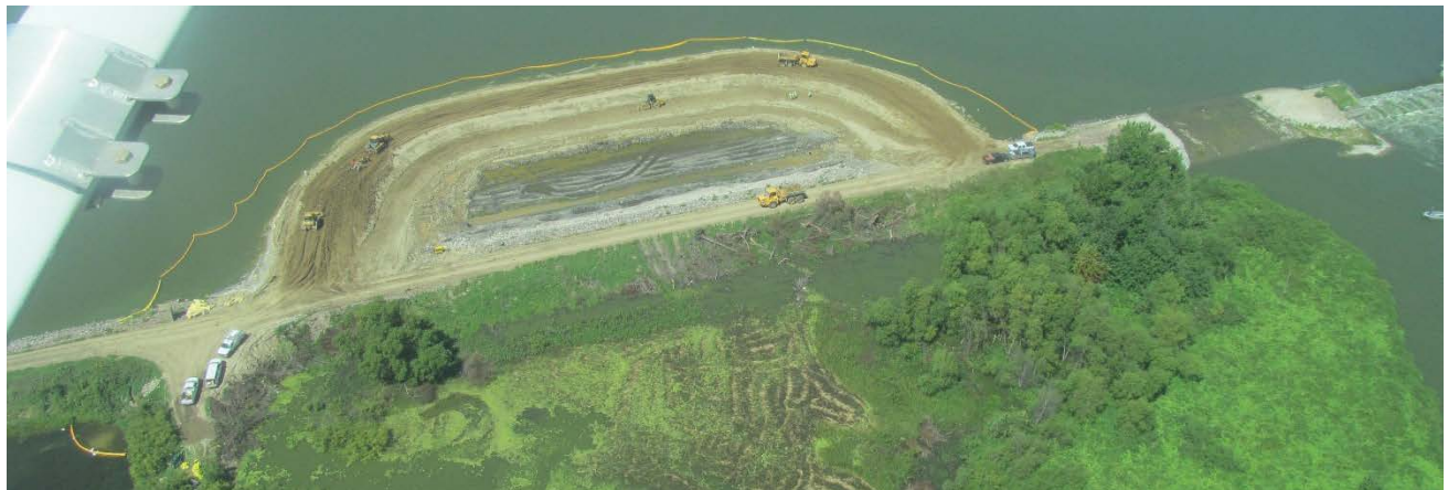
Figure 1 – Temporary cofferdam at location of future water control drawdown structure
