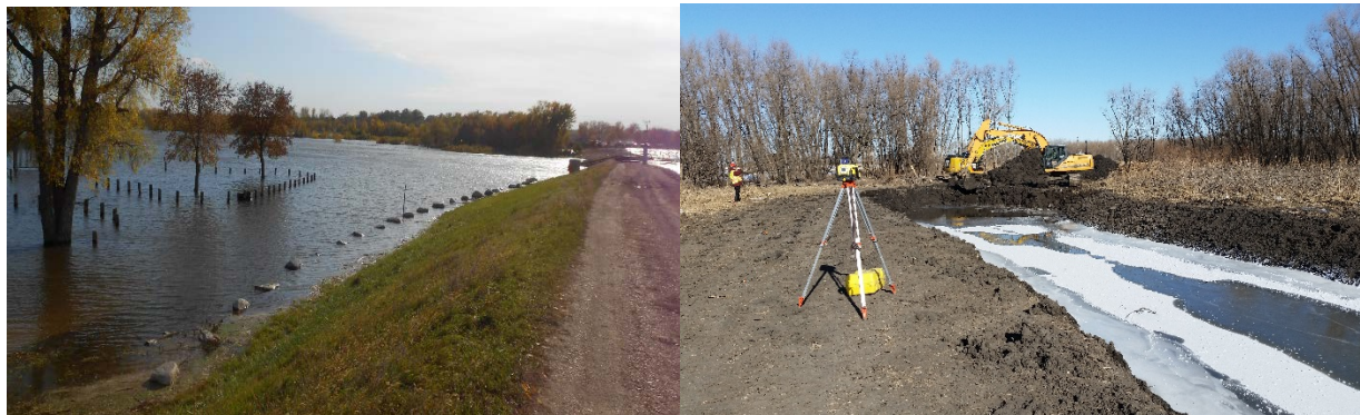
Figure 2- (Left) October 2017 flood event and (right) Pomme de Terre River channel excavation, January 2018.
