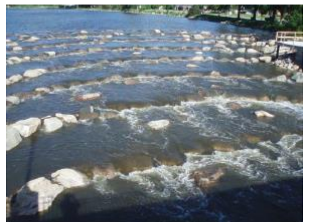
An arch-rapids, similar to what would be built to replace the Melrose Dam
