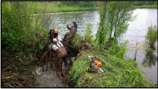
Beaver dam removal
