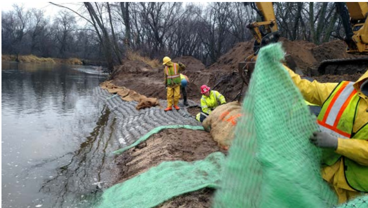
This is the above site part way through the repair of the erosion showing how the Flex-a-mat material is installed
