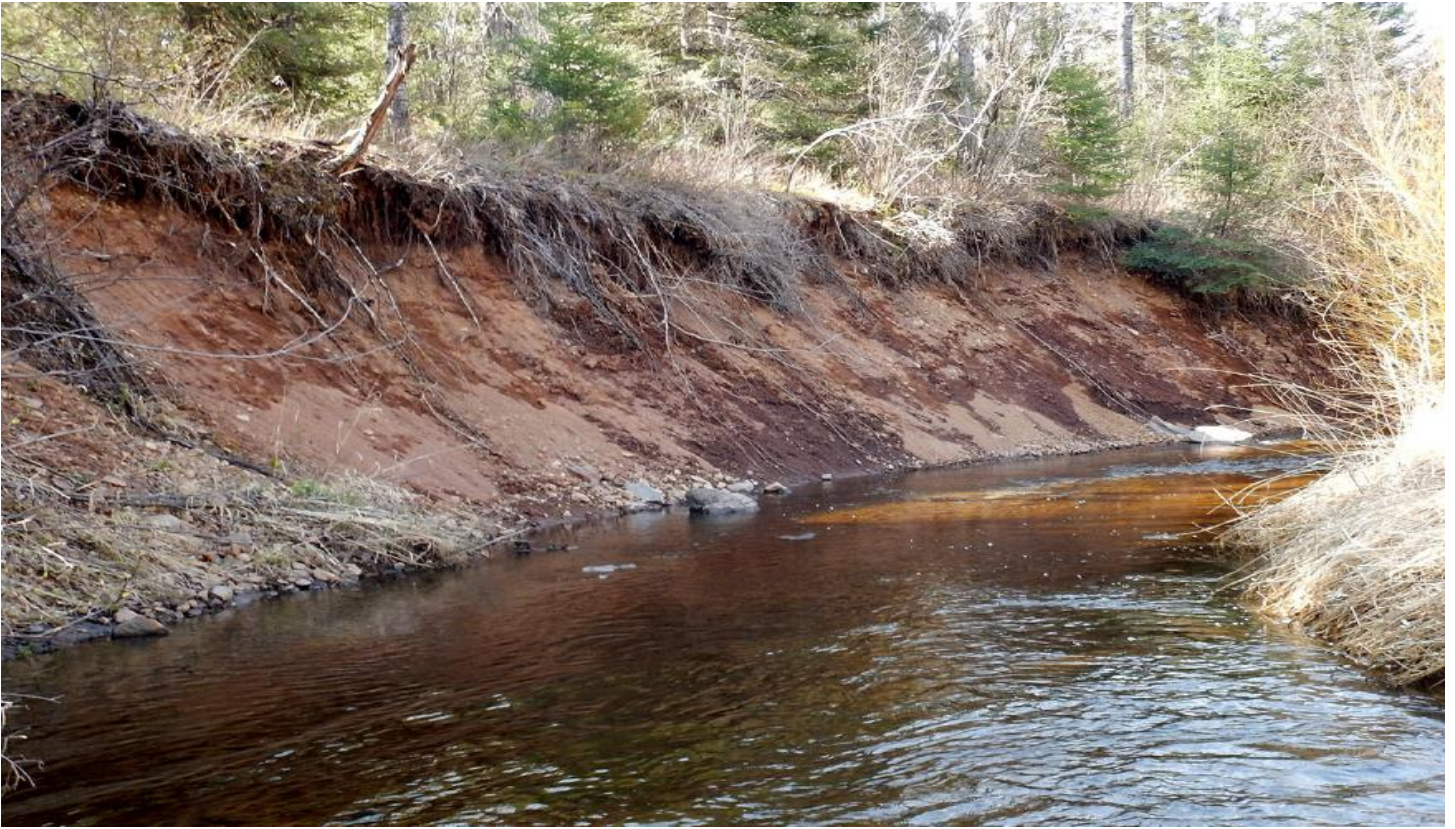
Reach 4 Eroding Streambanks
