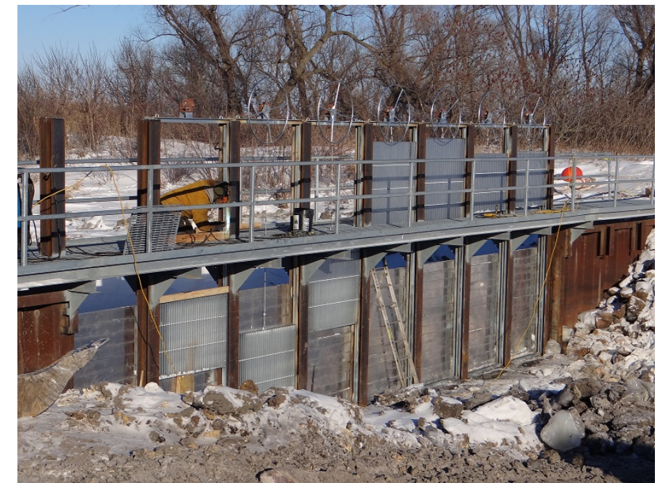
OHF-funded structure under construction at Swan Lake.
