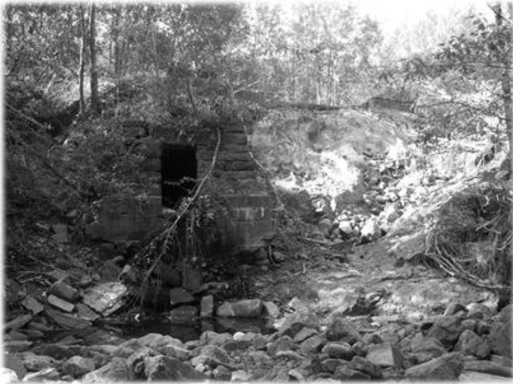
Downstream End of Culvert
