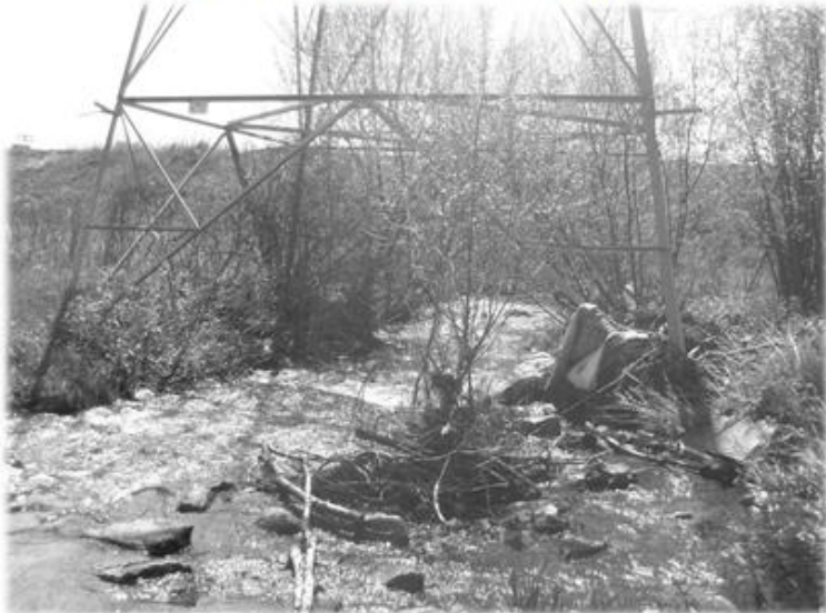
Electrical Tower in Stream Channel
