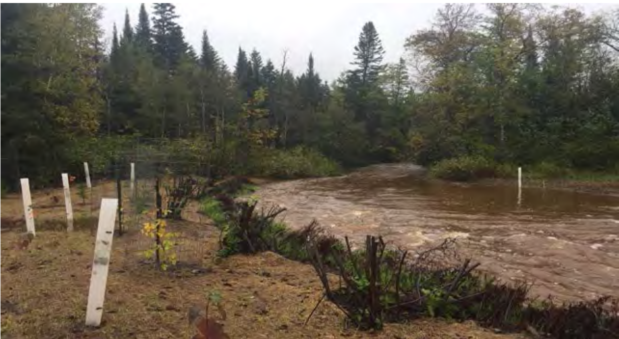
Figure 4 - Representative image of toe wood (near bank) and onsite transplants (near bank) along with the tree and shrub plantings with browse protection.
