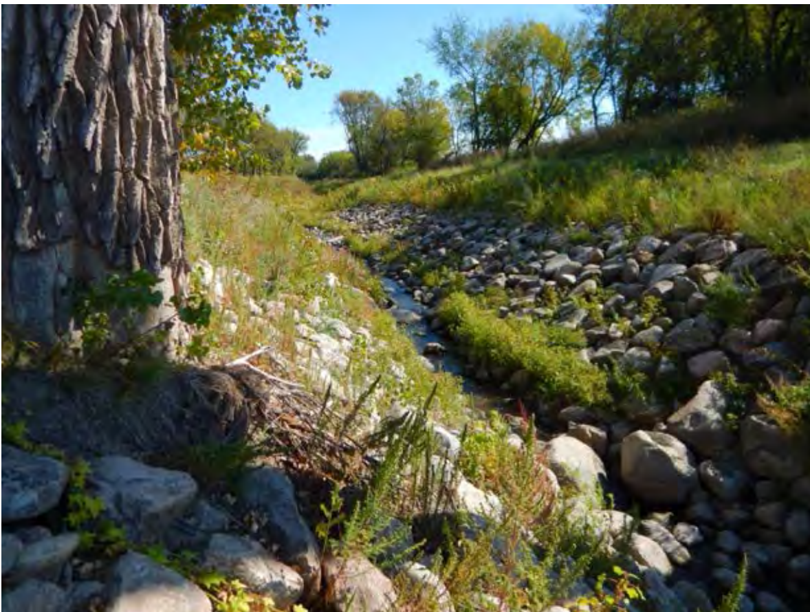
SR Photo 36: V Channel immediately upstream of confluence with the Red River. Note scour at base of cottonwood tree at top of slope.
