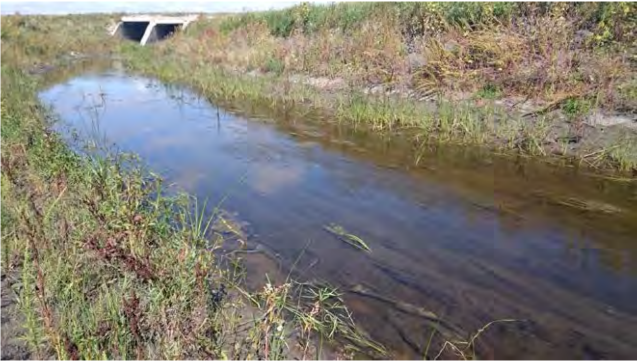
SR Photo 18: Stream channel upstream of the road crossing at 130th St. NW.
