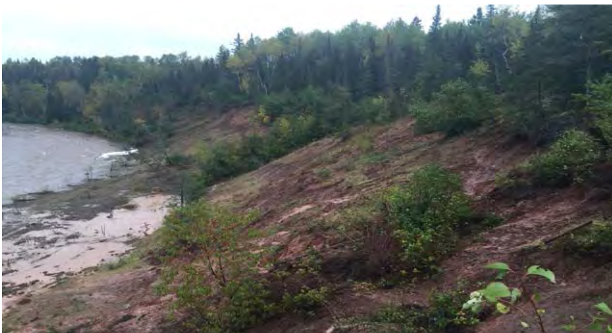
Figure 6 - Representative image of stabilization (bluff). As visible in photograph the attempt to establish vegetated cover on the clay bluff in question (right side of image) via hydroseeding is showing early signs of failure. It is acknowledged though that the primary project means for reducing sediment from the bluff is the realignment of the stream away from the bluff and the creation of a stable bluff toe and associated bankfull bench.
