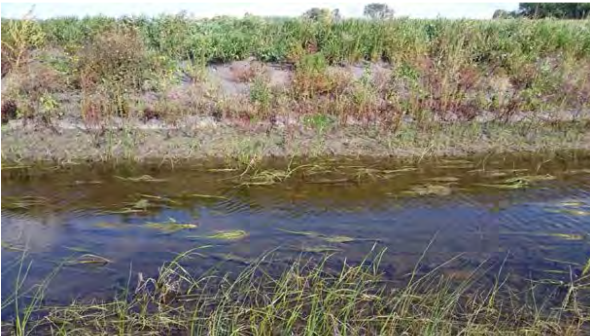
SR Photo 15: Bare slopes where unseeded.
