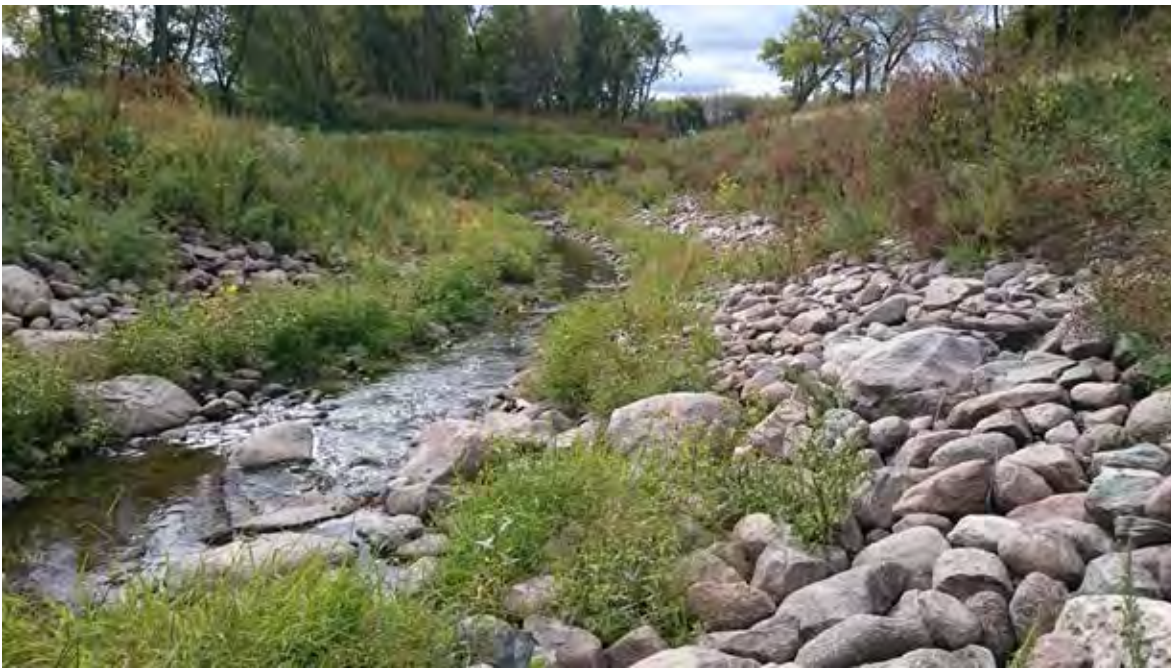
SR Photo 35: V Channel Riffle.
