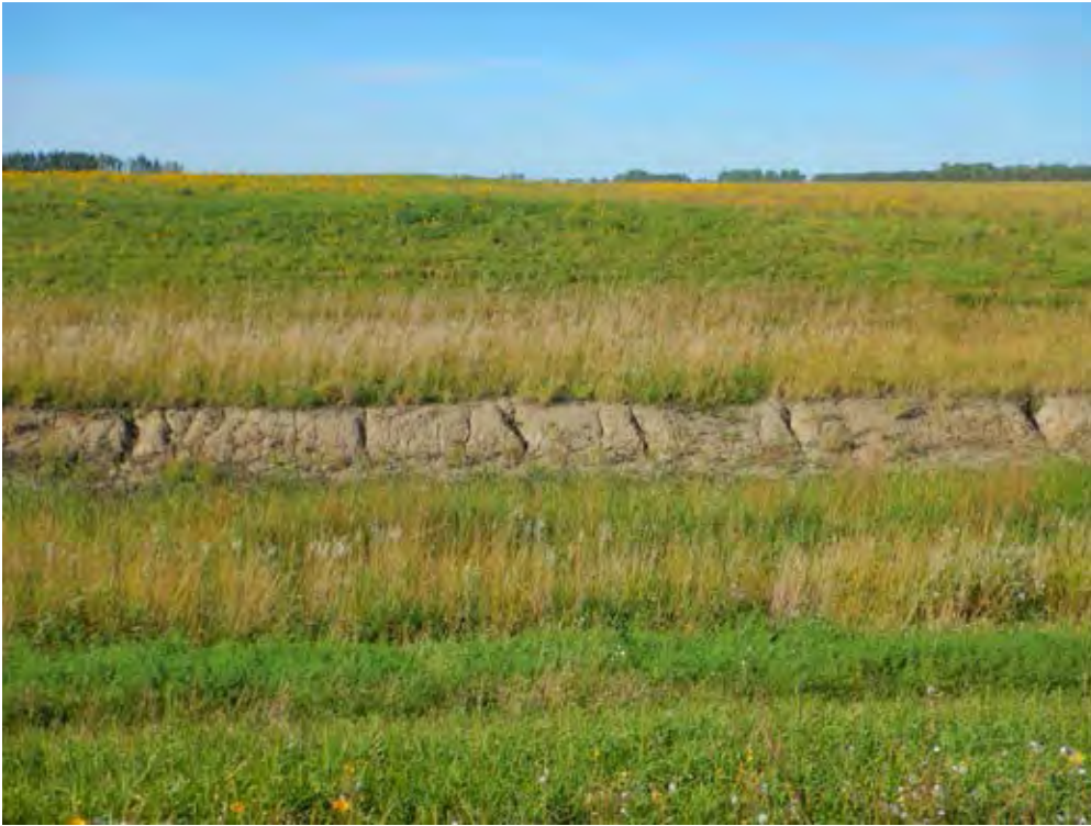
SR Photo 7: Constructed channel. Above
