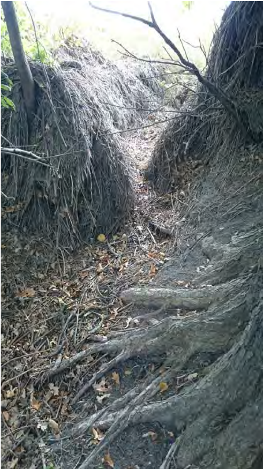
SR Photo 28: Gully above construction area in wooded area. Likely predates project as it is above existing exposed roots.
