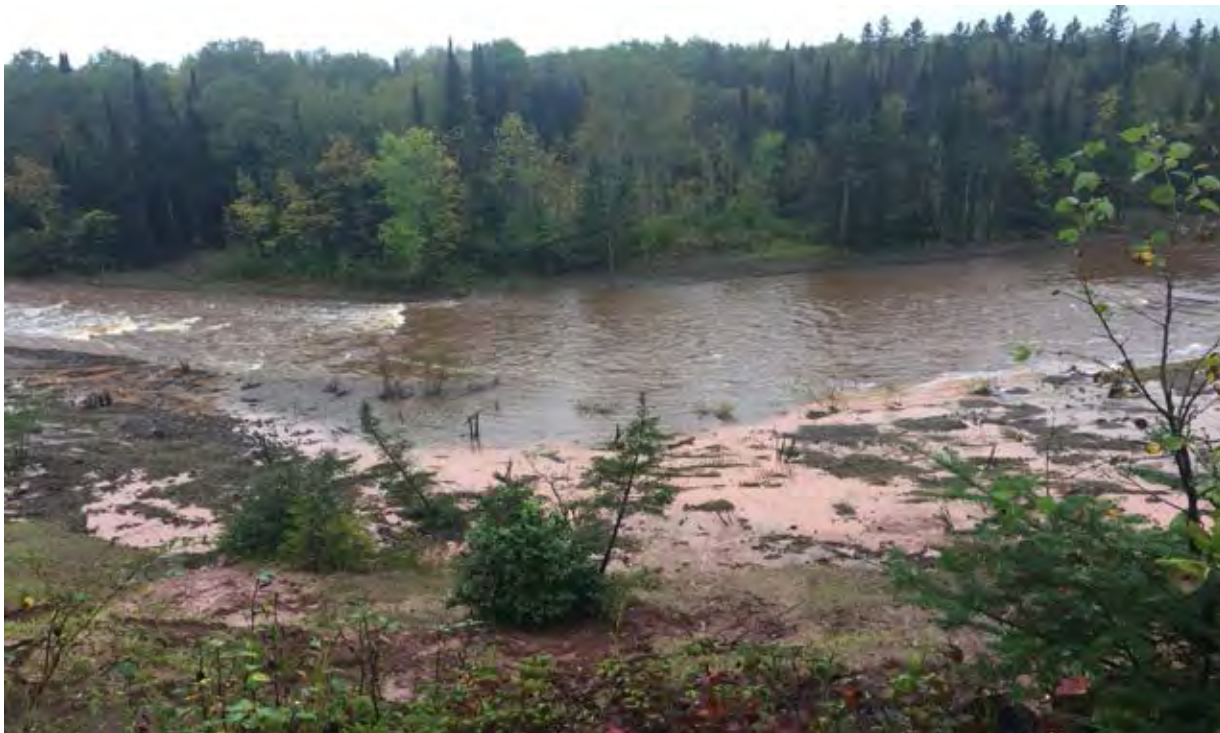
Figure 5 - Representative image of stabilization (bankfull bench). As illustrated in the photograph the created bankfull bench was appropriately being accessed (over-topped) by a near bankfull flow event.
