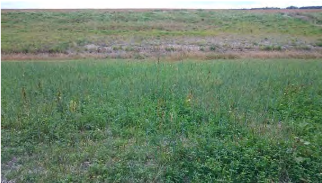
CC Photo 2: Stabilized slopes along upper channel. Note erosion at lower elevations near water level.
