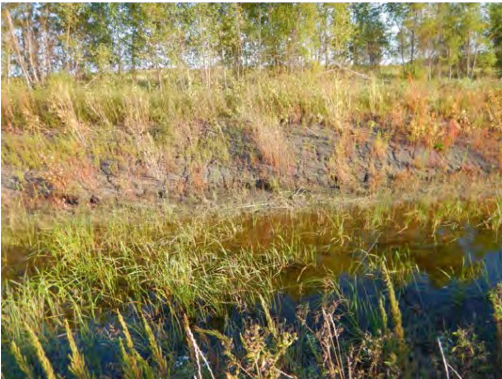
SR Photo 13: Unseeded slope at excavated channel.
